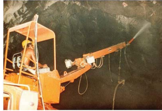
Fig 5: A truck mounted shotcrete robot
